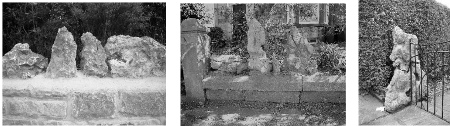
Plates 1a–c Water-worn limestone wall cappings (1a & b) and a gatepost (1c) in Lancaster
