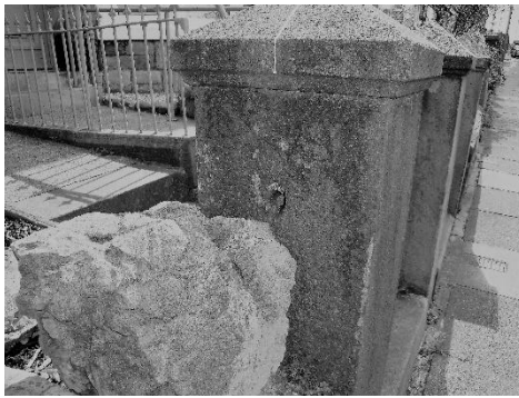
Plate 9 Evidence of limestone cappings having been installed after the railings had been removed
