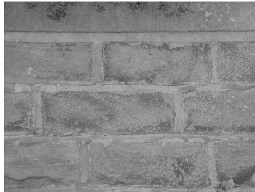
Plate 2b Rough-dressed (or Rock-faced)
