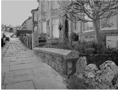
Plate 8 Evidence of railings having been removed
