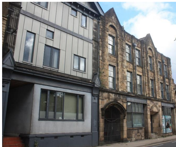
Fig. 6 The YMCA building and extension
