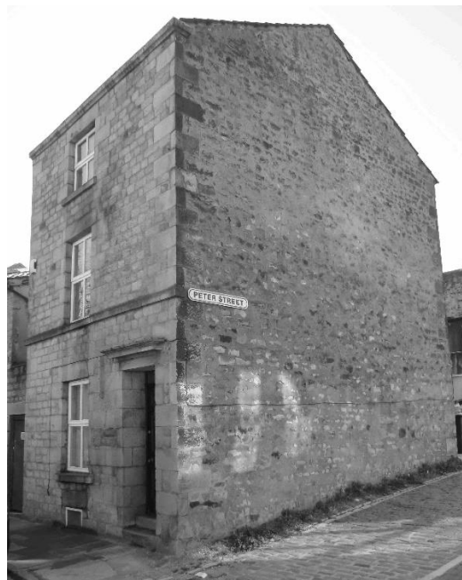
Fig.1 The single house on Peter Street, Lancaster, at the rear of St Thomas' Church, alleged to have been built by or for Peter Rogerson. In view of his later poverty this seems quite unlikely, but proof is lacking. Source: Andrew White
