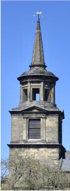
Figure 3: St John's bell tower North Road, Lancaster, 1782
